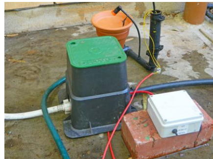
Place the terracotta saucer on the terracotta pot and adjust the control dripper
