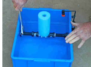
Tighten the two back-nuts
