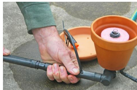
Connect the irrigation application to the outlet
