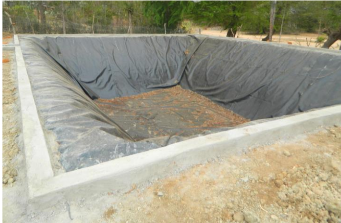
Farm pond in Kenya for gravity feed drip irrigation
