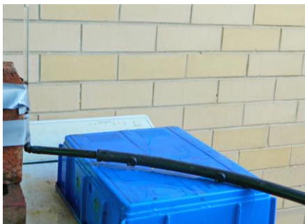
Zone 1 with 2 drippers at level -1.74 metres.
