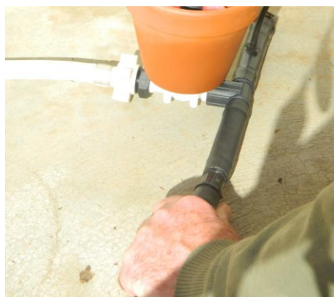
Connect the irrigation application to the 19 mm poly pipe
