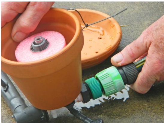
Connect the water supply to the valve inlet
