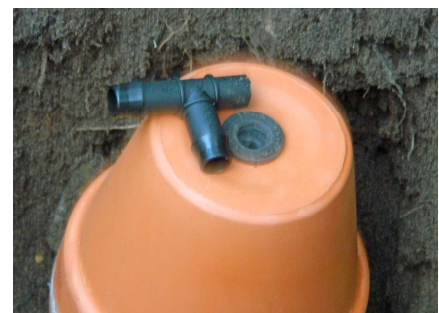
Step 4. Gently press the pots together and allow 24 hours for the sealant to cure
