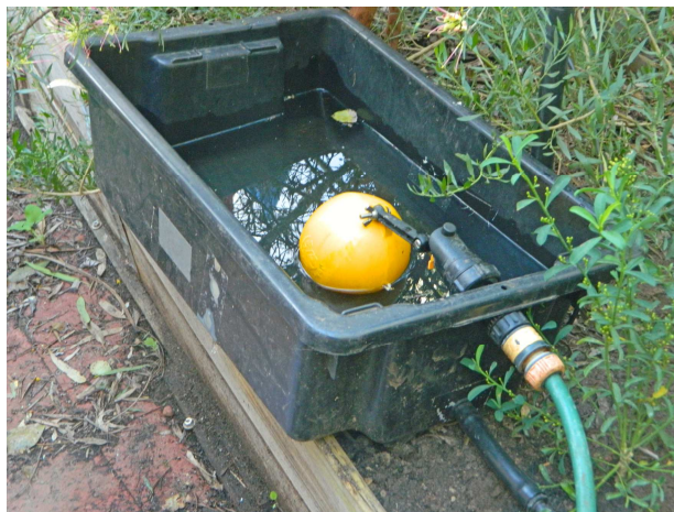
Polypipe network connected to the outlet of a storage container with a float valve
