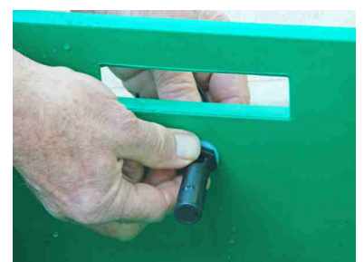
Install the float switch
