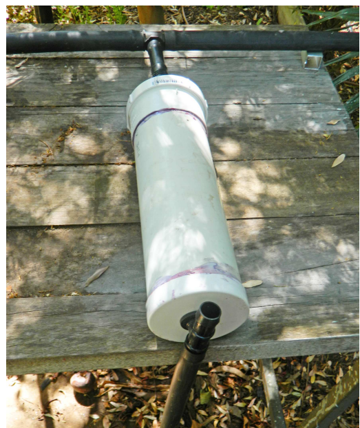
Dripper assembly installed showing the overflow outlet and the polypipe delivering water to the zone
