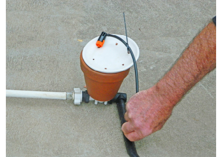
Connect the control dripper to the irrigation application
