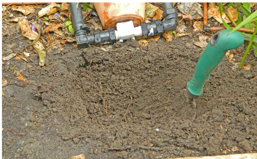
Step 1. Dig a hole midway between two adjacent plants. There should be no irrigation drippers near these two plants.
