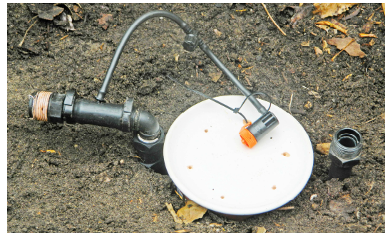
Step 2. Connect vertical pipes to the valve inlet and outlet and position the valve in the hole so that rim of the pot is above ground level. Back fill the soil around the pot. Connect the control dripper to the outlet pipe.
