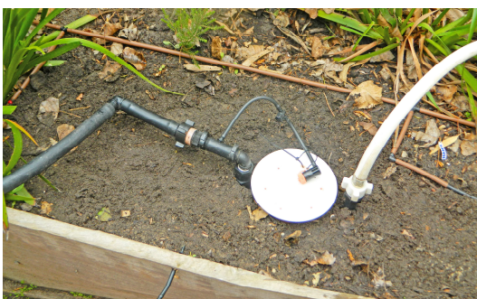
Step 3. Connect the water supply to the inlet pipe and connect the irrigation application to the outlet pipe.
