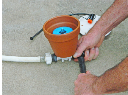
Connect the irrigation application to the valve outlet
