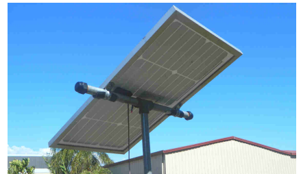
Solar panel mounted on a pole
