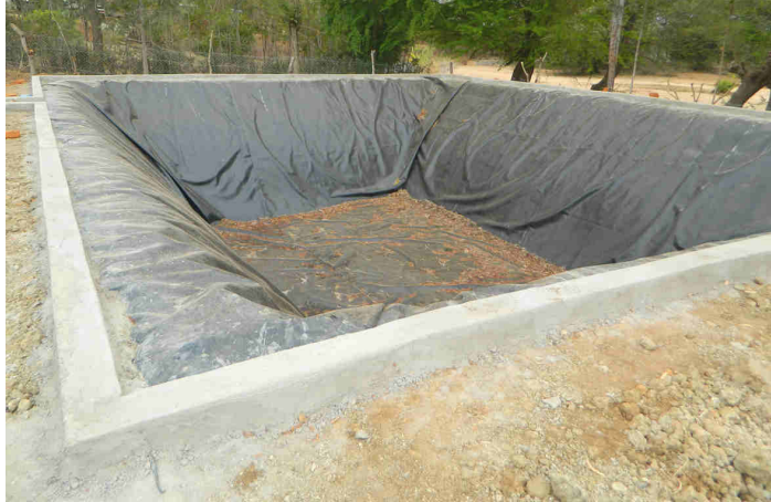
Farm pond in Kenya for gravity feed drip irrigation
