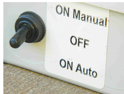
Pump controller with the switch in the ON Auto position
