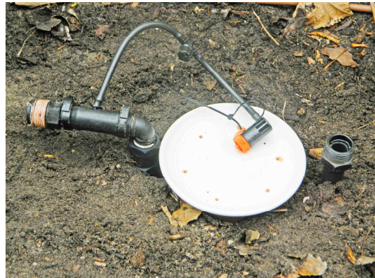
Step 7.2. Adjust the inlet and outlet pipes so that they are vertical. Position the controller in the hole so that rim of the pot is above ground level. Back fill the soil around the pot.
