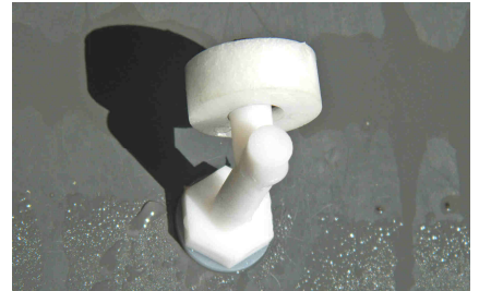
Float switch on the inside of the header tank with the float shaft pointing up
