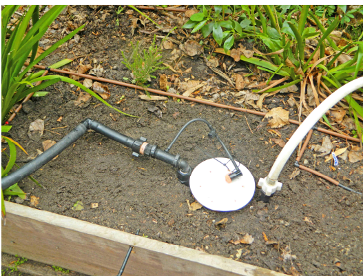
Step 7.3. Connect the water supply to the inlet pipe and connect the irrigation application to the outlet pipe.
