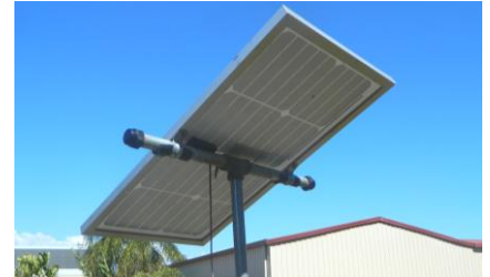
Solar panel mounted on a pole
