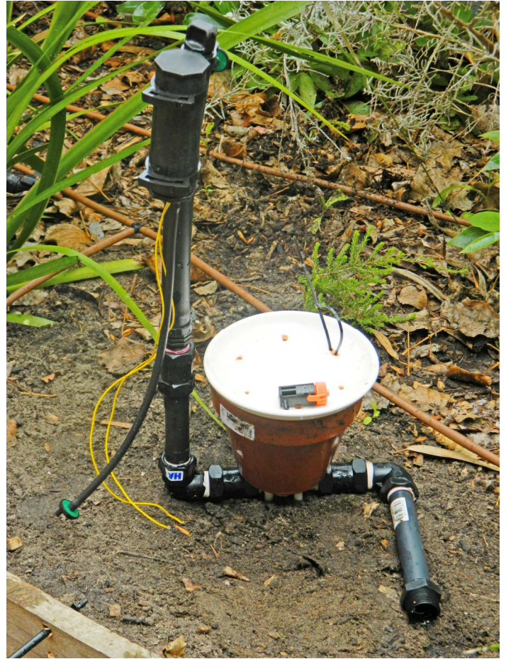
Above ground installation of the Terracotta Irrigation Controller
